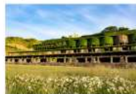
KITAZAWA FLOTATION PLANT
